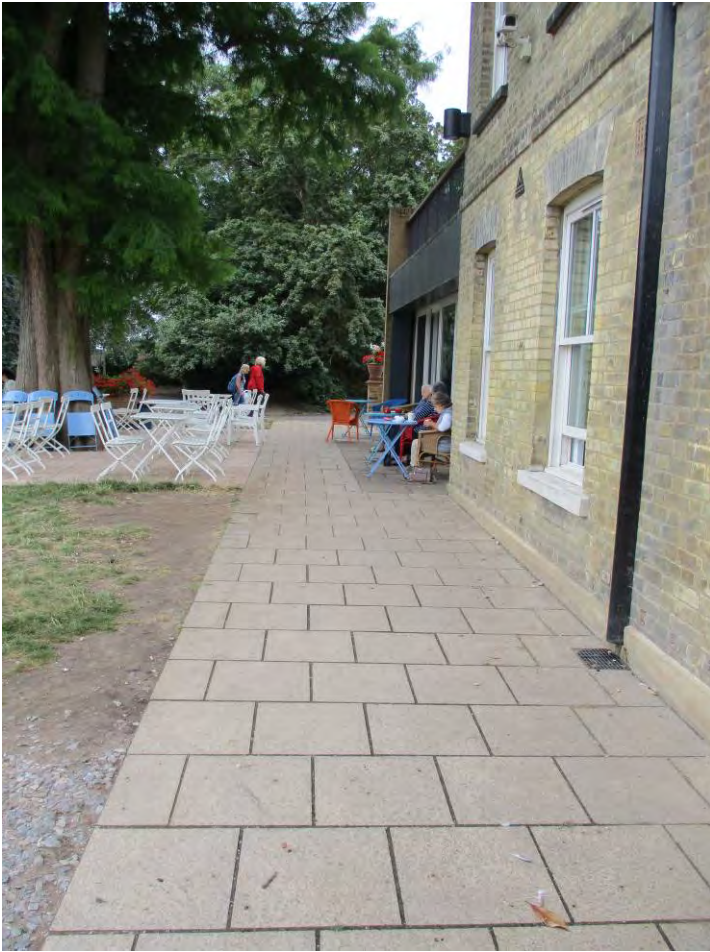
Existing path in front of West House – looking South
